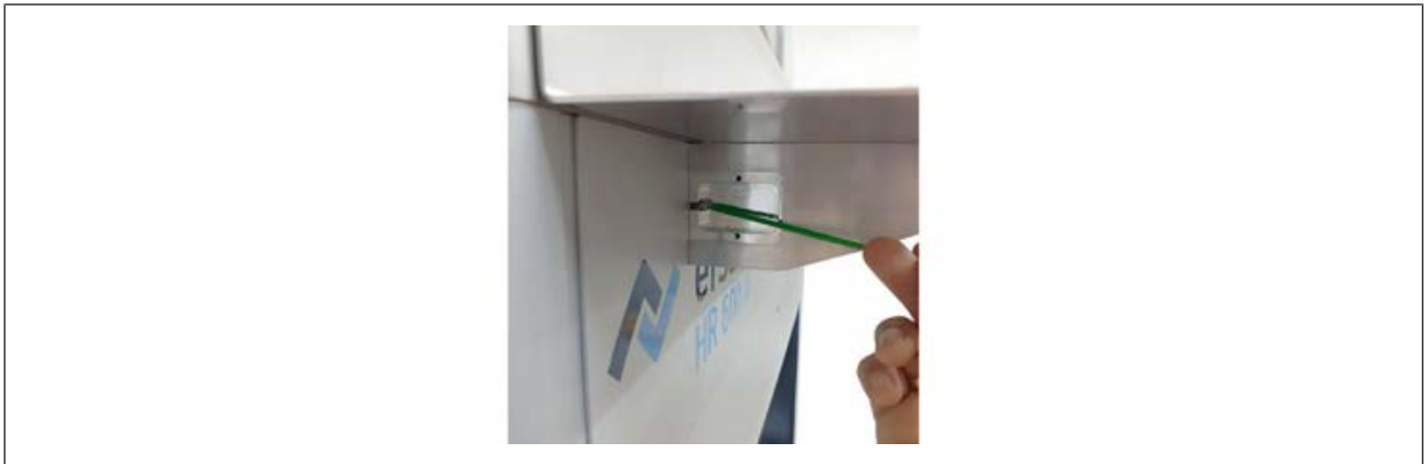
Fig. 20: Screwing the supports on
