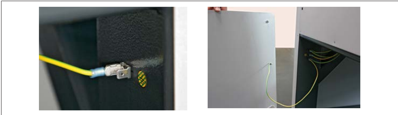
Fig. 12: Connecting an earth cable
