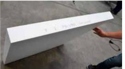
Sorted panel stacks according to construction plans: inclined roof panel with number and gradient.
