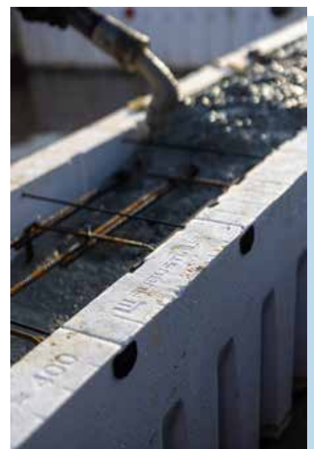
The U-shaped formwork element in use during the pouring of a foundation
