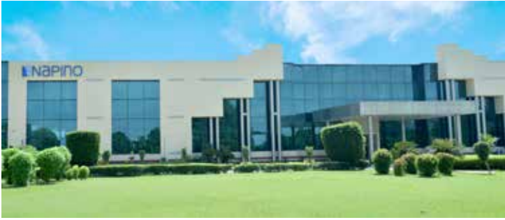
Napino headquarters in Manesar; source: Napino
